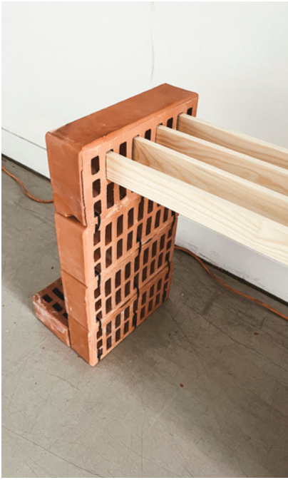
22. Prototype No. 1 – Detail of setting of scantlings in brick holes
